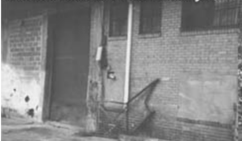
The Finders' warehouse in northeast Washington, DC.
